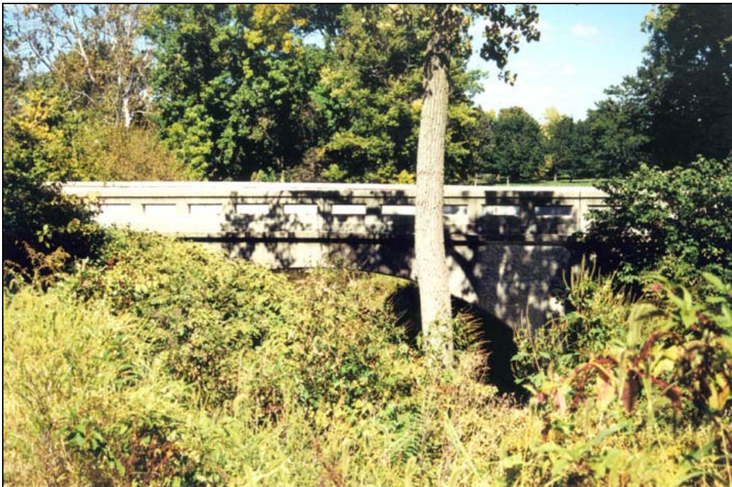
Figure IV.12 1923 filled-spandrel arch bridge on Pagoda Drive spanning a densely vegetated section of Bean Creek. (R-IV-17-HL.jpg)
