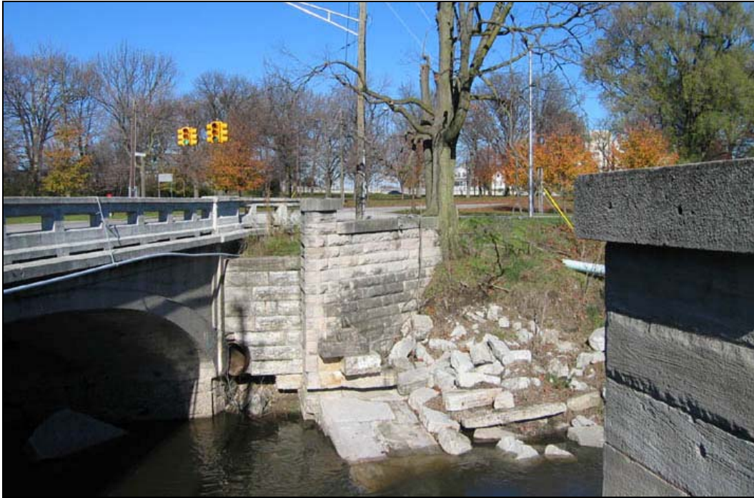
Figure IV.13 Rebuilt 1928 filled-spandrel arch bridge with original stone wing walls and rectilinear concrete railings crossing Pleasant Run. Remnants of the old dam are visible in lower center of photograph. (R-IV-119_1954.jpg)
